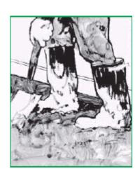
Concrete, like all other materials, will slightly change in volume when it dries out. In typical concrete this change amounts to about 500 millionths. Translated into dimensions-this is about 1/16 of an inch in 10 feet (.4 cm in 3 meters). The reason that contractors put joints in concrete pavements and floors is to allow the concrete to crack in a neat, straight line at the joint when the volume of the concrete changes due to shrinkage.
